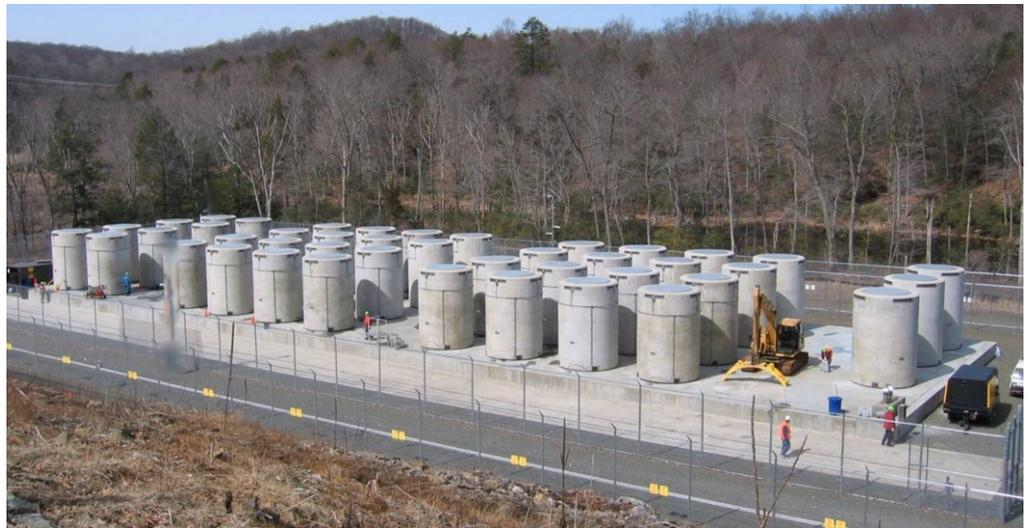
Before used fuel is loaded from a pool into a canister, the canister is lowered into the storage pool inside a shielded transfer cask. If the fuel is to be loaded into a metal cask with an open basket, the cask is lowered into the pool with the basket installed. Following loading of the fuel, a lid is installed and the cask is removed from the pool. The water is drained from the cask and, if a canister is
