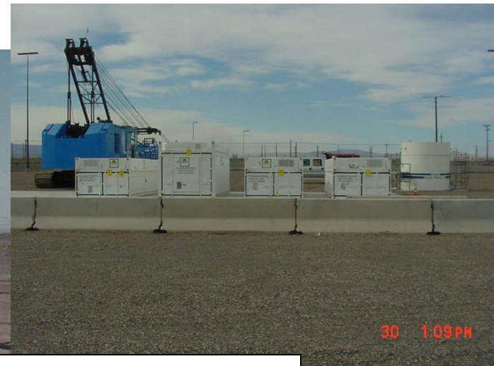
Far Left: Cask placement at ISA. Center: TRIGA Rad-Vault lid installation;. Far Right: NAC-1 Casks in ISO (standard) Containers
