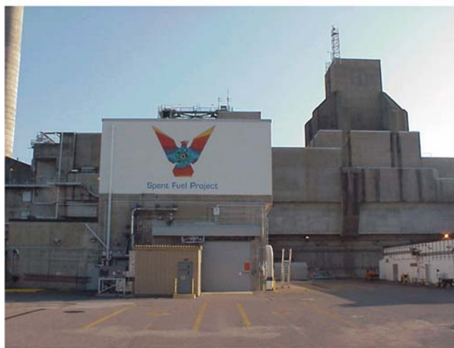
Figure 2. L Basin Building (from Hixson 2015).
