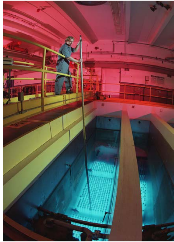
Figure 1. Pool Storage of Cesium and Strontium Capsules at the Waste Encapsulation and Storage Facility at Hanford (Gephart 2003).
