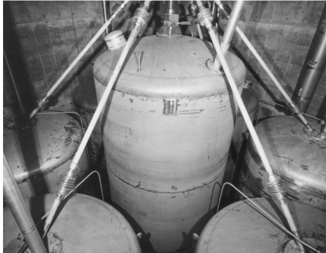
Figure 2. Storage Bins in CSSF III. The Center Bin is Surrounded by Six Shorter Bins (Staiger and Swenson 2018).
