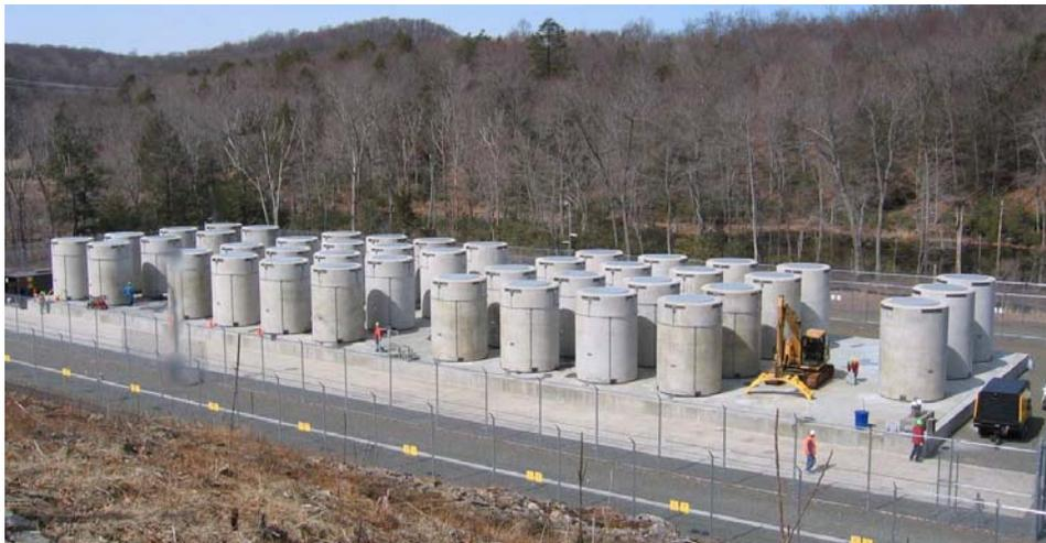
**Figure 3. Independent Spent-Fuel Storage Installation**
